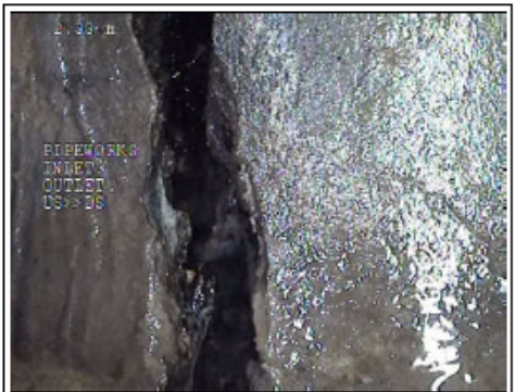
Cracking Circumferential, Large, from 12 to 12 o'clock, (CC,IP,OT).
