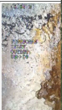
Joint Faulty, Large, f (STAINING,IP).
